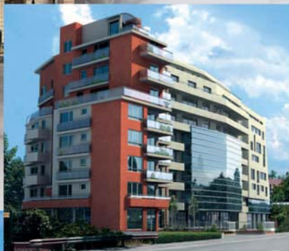
9-storey res. bldg., Vitosha, Sofia
