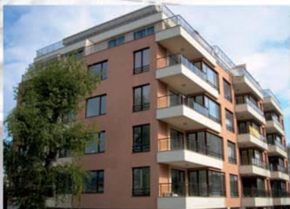
7 storey res. bldg., Vitosha, Sofia
